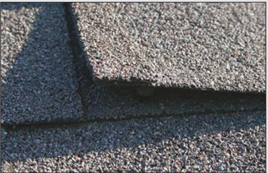
Nail Pop – An elevated nail that can push a portion of the shingle off the roof plane. Over time, this pop can cause a hole in the shingle.
