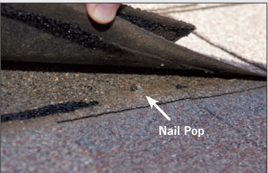
Nail Pop – An elevated nail that can push a portion of the shingle off the roof plane. Over time, this pop can cause a hole in the shingle.
